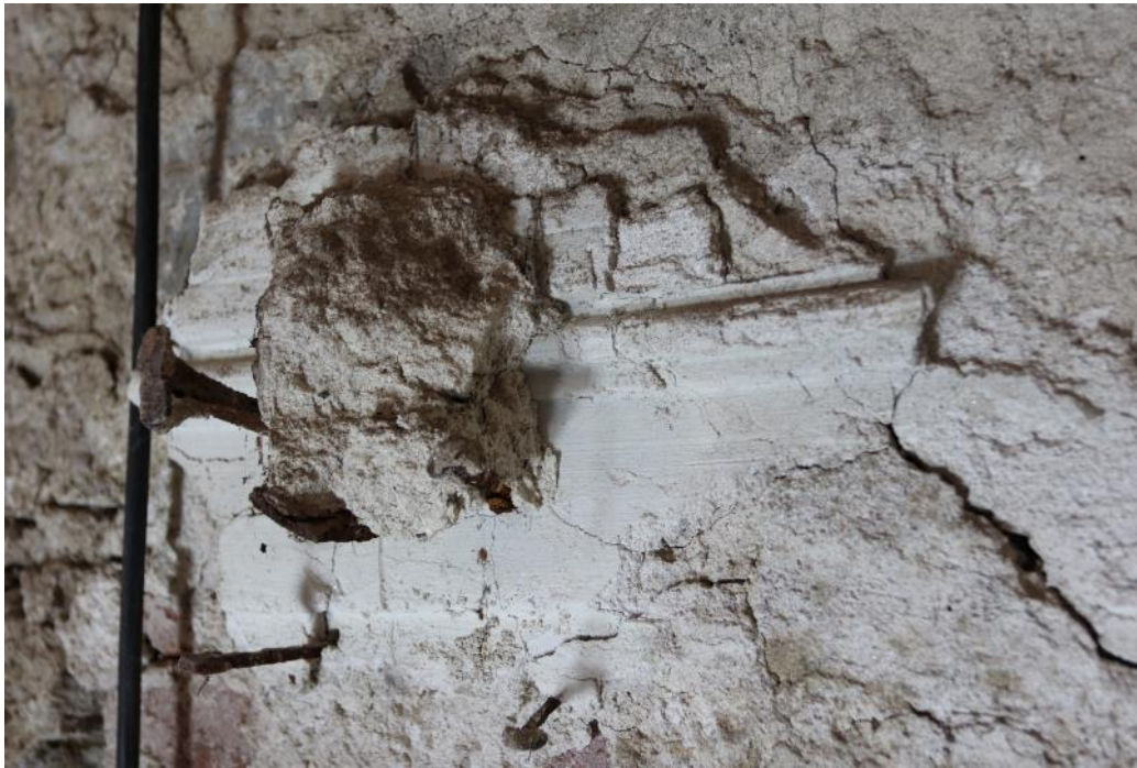
Brick support structures of architectural stuccoes, first layer of arriccio
